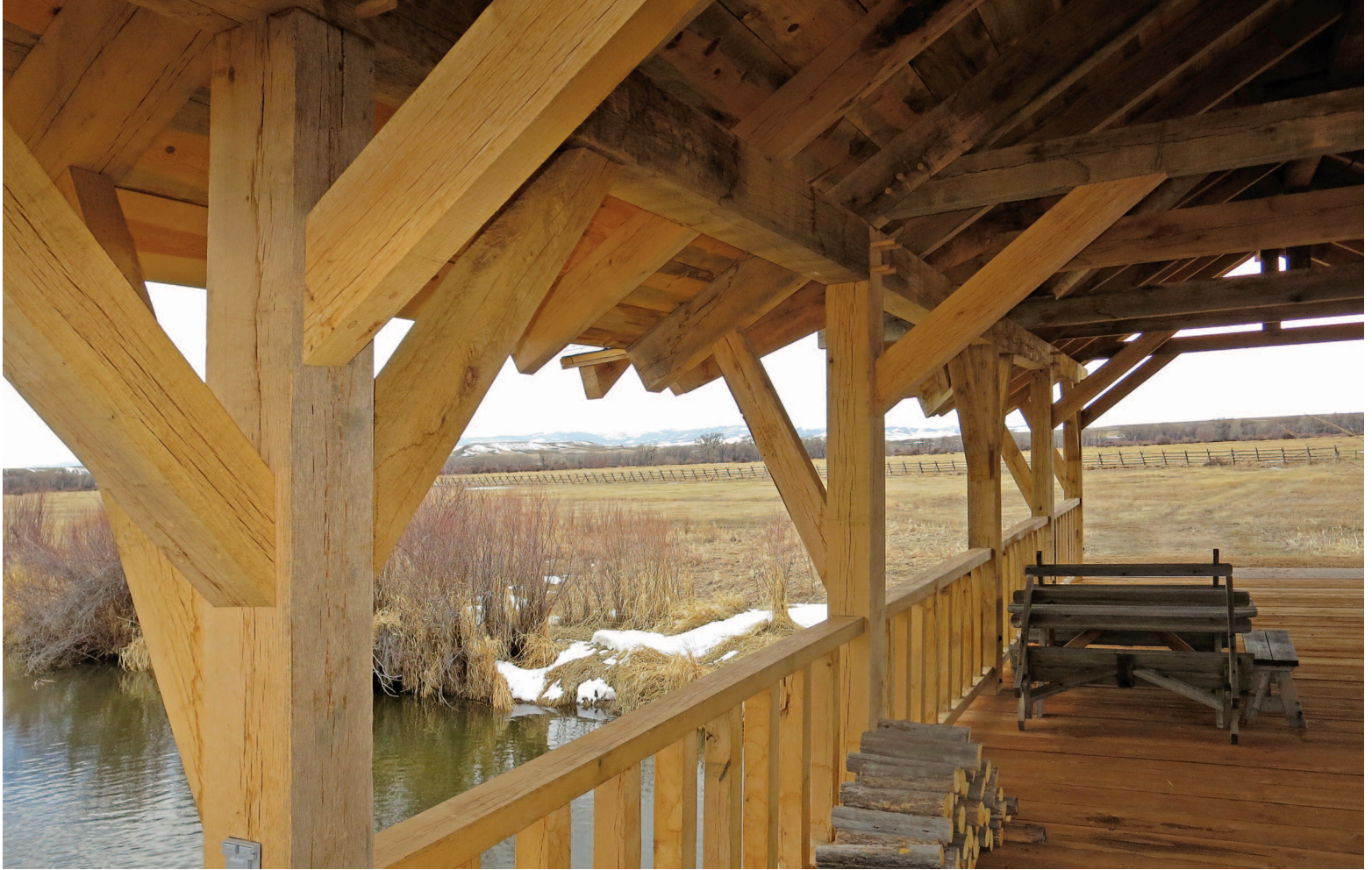
White oak framing timbers grew in Maryland. Mortise and tenon joinery, with braces, valleys and jack scribed, butted and fastened.
